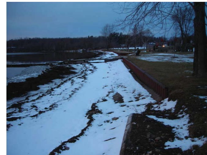
Figure 6. Steel sheet pile shore protection in Centennial Park
